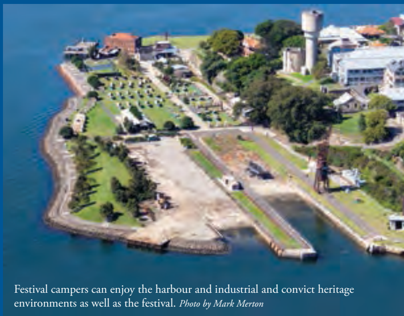
View of Cockatoo Island industrial heritage buildings and equipment. Photo by Dragi Markovic
